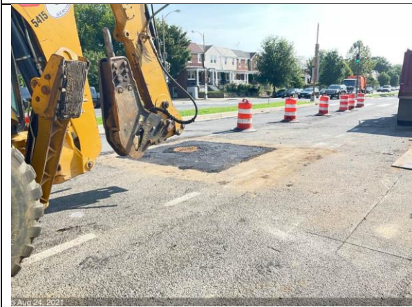
1800 Block C St NE– M6-10 cover and tempoary asphalt
