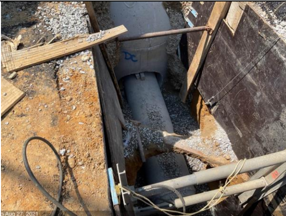
1800 Block C St NE- 18" RCP between M6-3 to M6-4
