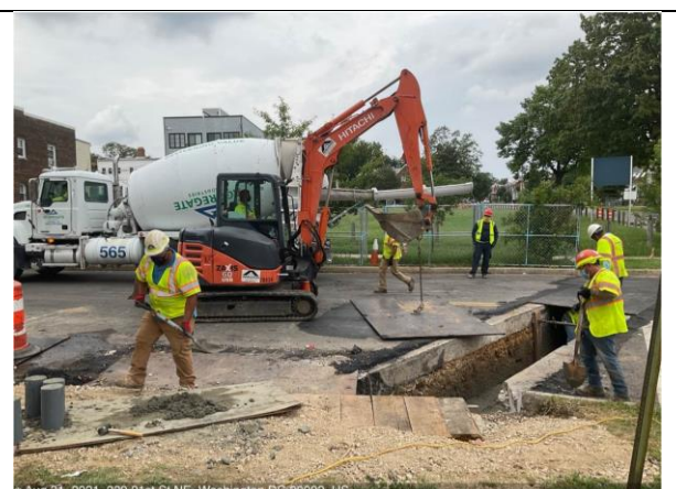
C St NE & 21st St – 15" RCP cradle between M8-4 and I8-7
