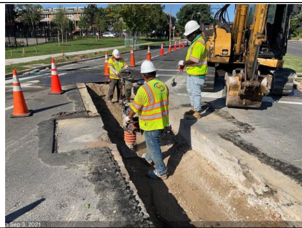
C St NE & 18th St – Backfill 18" RCP between M6-3 and M6-4
