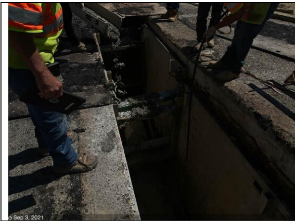
C St NE & 19th St – Place concrete for 15" RCP cradle between M6-10 and I7-3
