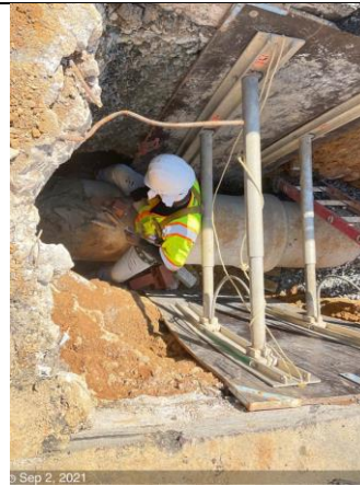
C St NE & 18th St – Place 18" RCP between M6-3 and M6-4
