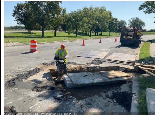
C St NE & 21st – 15" RCP backfill between I8-7 to M8-4
